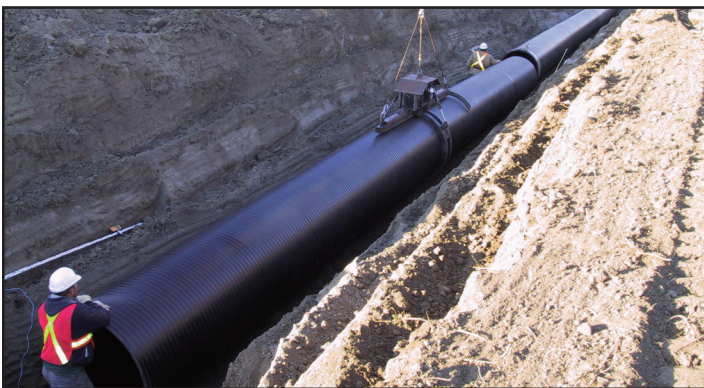
48" Dia. Weholite Pipe: Long Pump Canal
