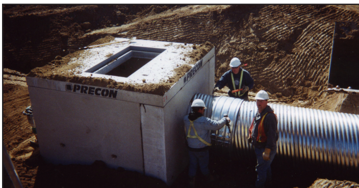
Precast Drop Structure to John Ware Canal
