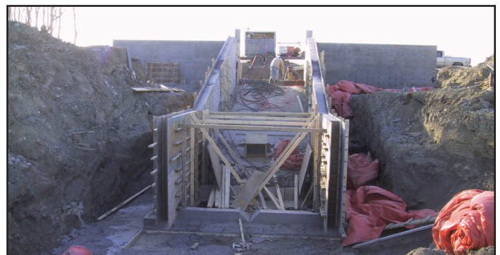
Cast-in-Place Check Drop: Sec. G Springhill
