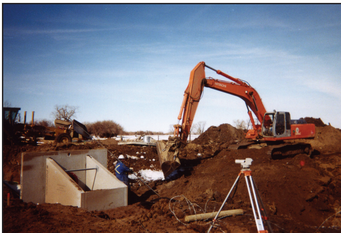
Lateral Turnout Structure: Lower North Branch Canal
