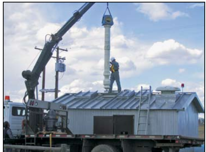
Upgrading Pumps on Long Pump Lateral
