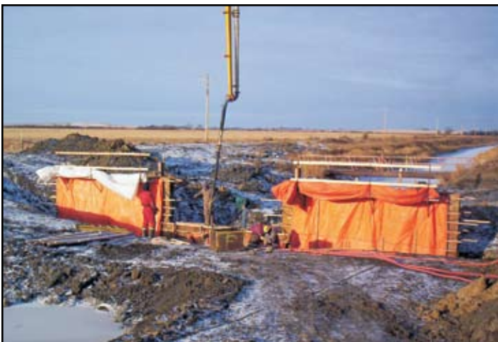
One Tree Check Structure
