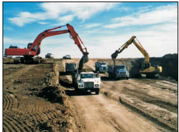
Construction of North Bantry Stilling Pond
