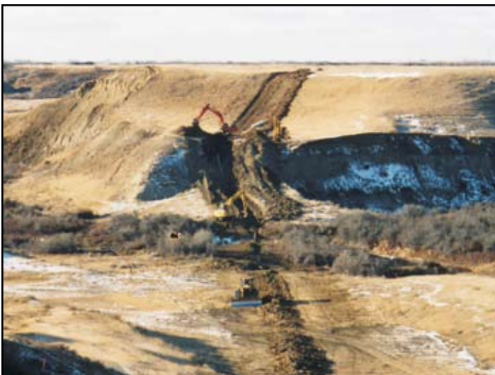
R North Bantry Pipeline
