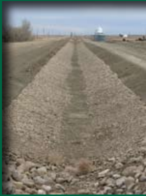
X Tilley: Gravel on poly liner.
