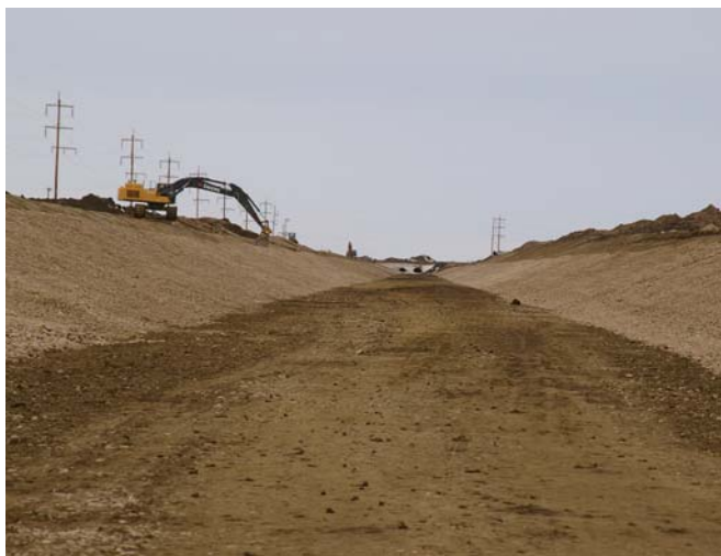
Armour Placement on Side Slopes - Kitsim Feeder
