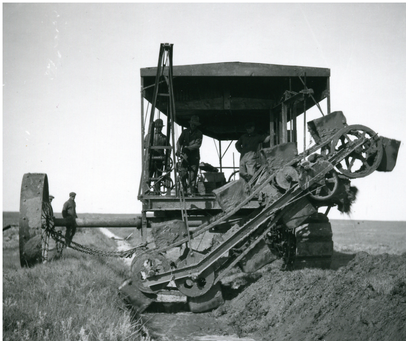
Canal cleaning with a Ruth Dredge September 1919.
