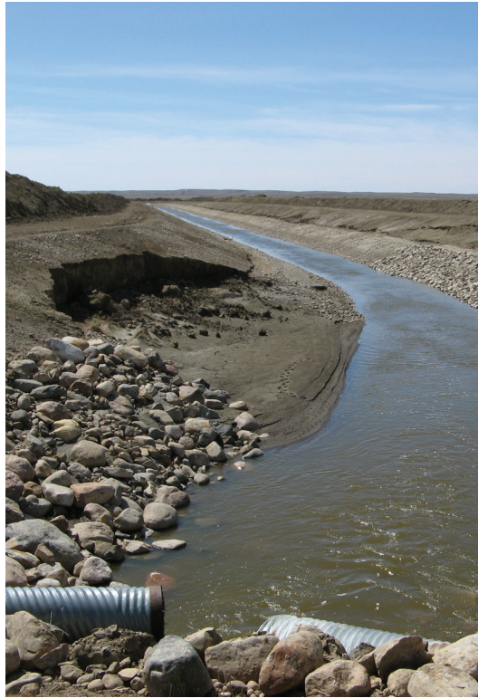
Erosion damage on John Ware Canal due to heavy spring runoff.
