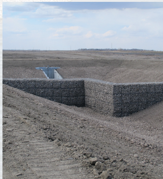
Stilling pond construction.
