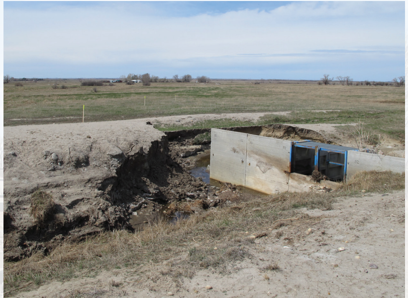
Washed out structure on AH North Bantry.
