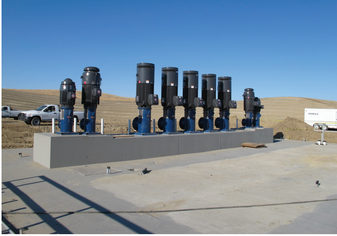
Pumps at the Rolling Hills Reservoir acre development pump station.
