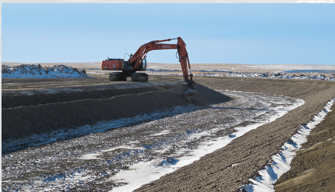
Placing armour on North Bantry.
