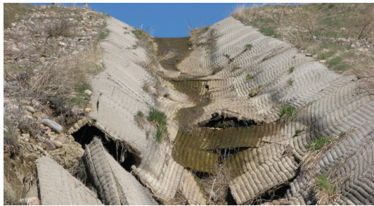
Bow Slope spillway washout.
