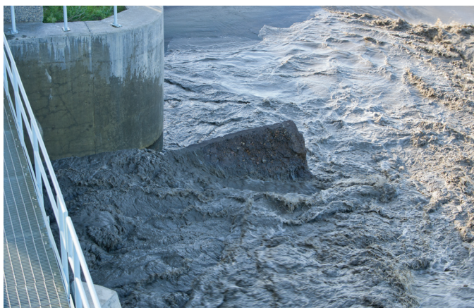
Bassano Dam: Damaged caused by high flows
