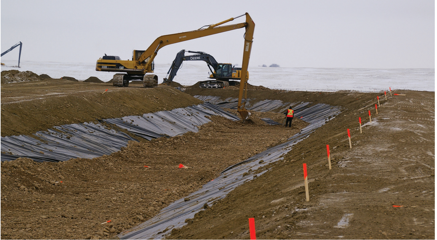
Antelope Creek Canal Placing armour on plastic liner
