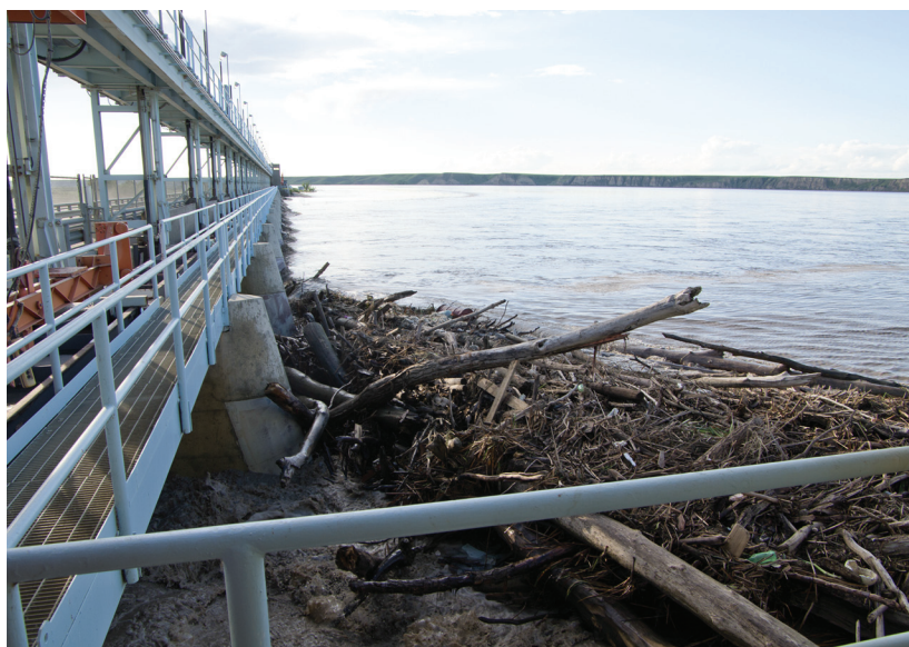
Bassano Dam: Trash backing up in front of gates 1, 2 and 3
