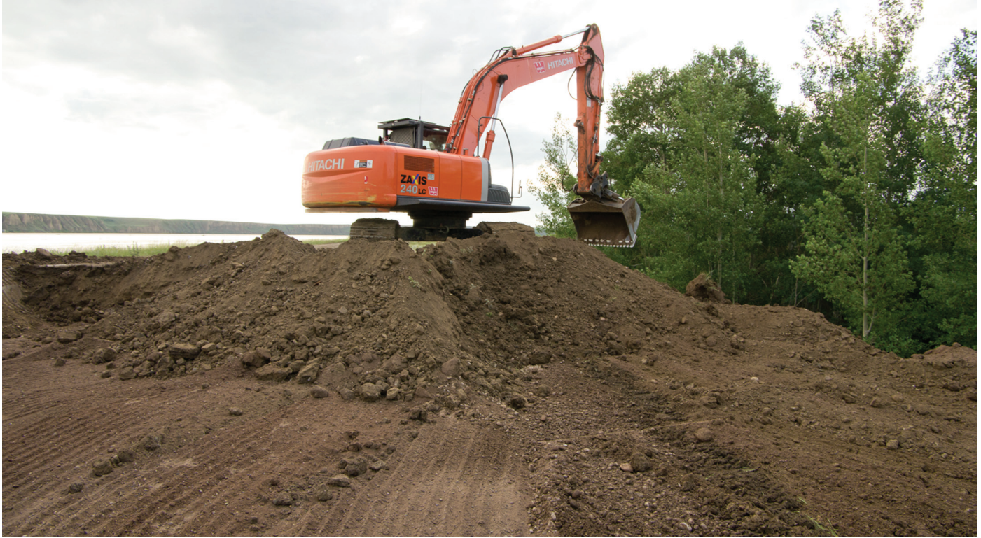
Bassano Dam: Removing the clay top from the fuse plug
