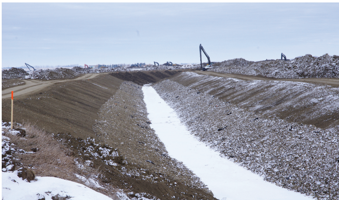
One Tree Canal Armoured
