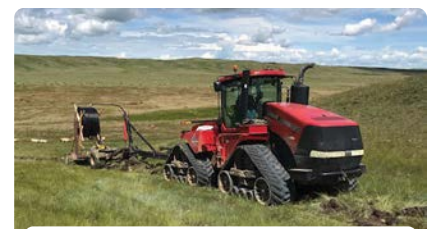
Installing Grazing Waterline
