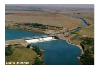
This major facelift cost 14 million dollars with the end result being a very modern dam capable of diverting 100 m<sup>3</sup>/s (3,500 cfs) into the District's water system.
