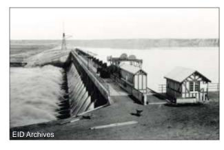
On the north end of the spillway an earthen embankment was constructed to help contain the river. This embankment was 14m (45 ft) high, 2200 m (7,000 ft) long and required 3,000,000 m<sup>3</sup> (10,000,000 ft<sup>3</sup>) of fill material to construct.
